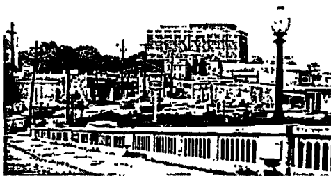
The view from the overpass c. 1950.
